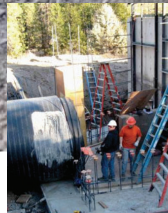
Weholite pipe being prepared for joining.
